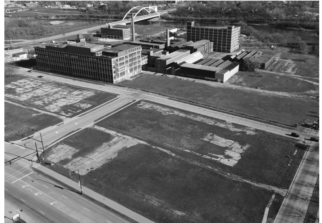
Site's Current Condition
